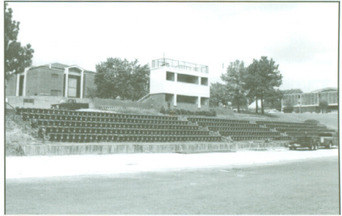
Permanent seats were installed in August '99 at Monarch Field.
