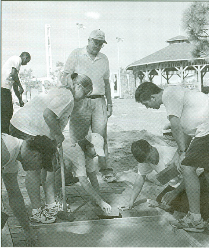
Dr. Hendricks and volunteers for this spring's "Show You Care Day" project install brick walks at Fannie Farmer Memorial Park.
