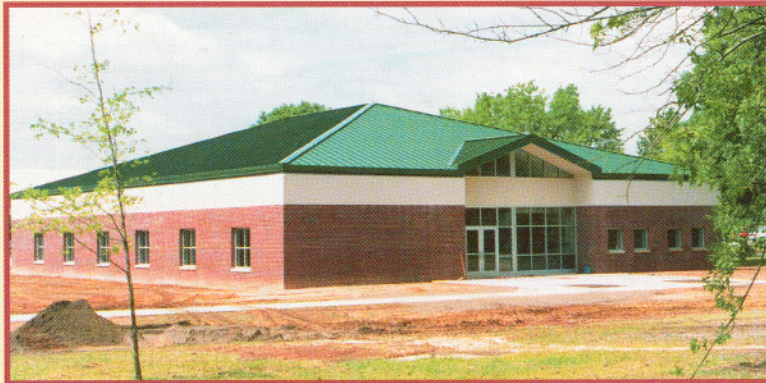
Math & Computer Science Building
