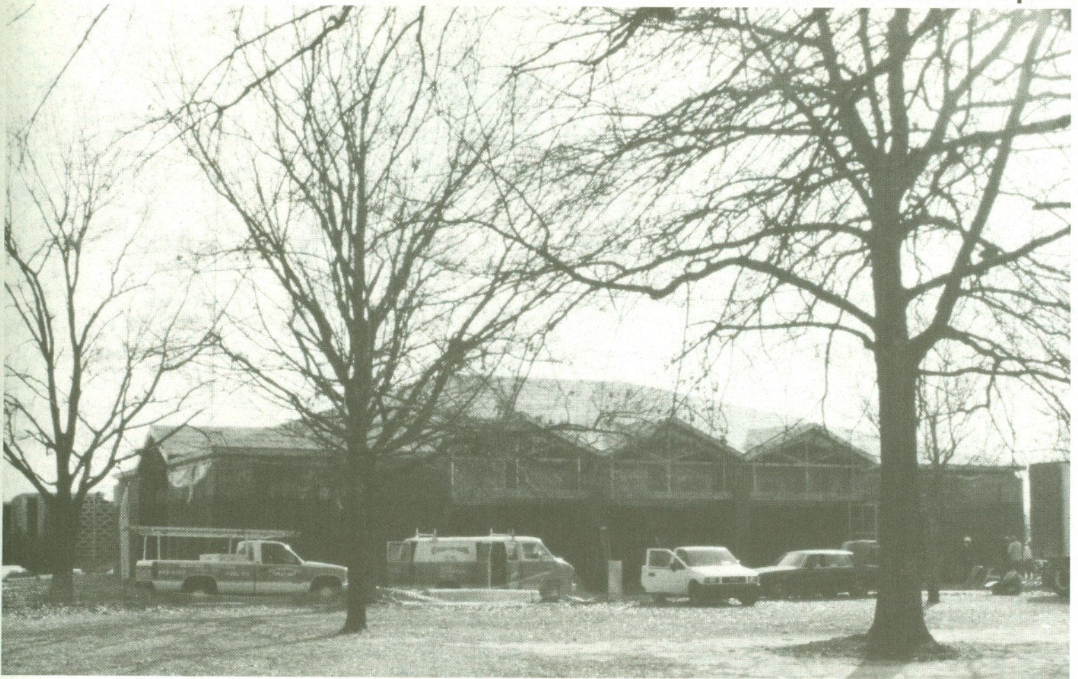
The groundbreaking for the new Math and Computer Science Building took place in October. It will open this summer.
