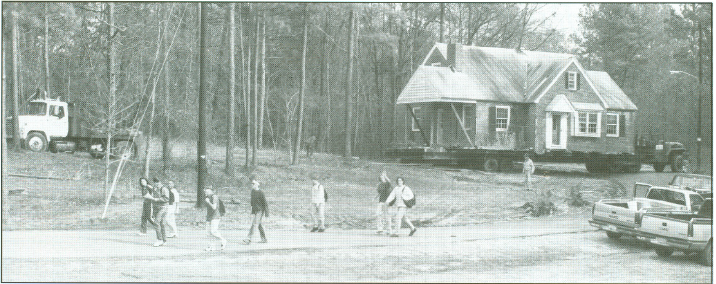
House movers maneuver the old Taylor residence into a clearing behind Cumberland Hall. The house will be renovated to serve as a student lounge/snack bar.
