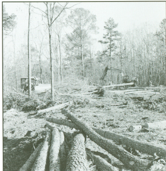
Bulldozer clears trees for second half of college golf course.
