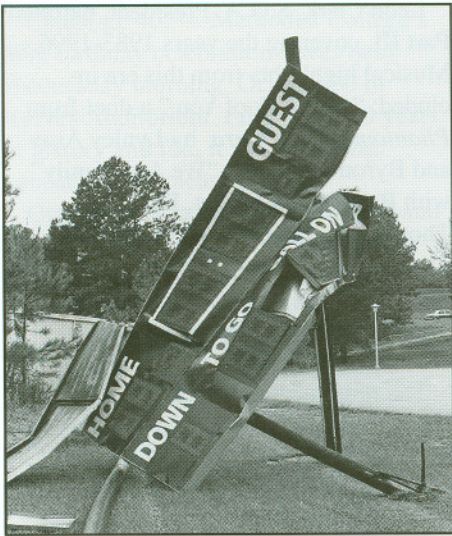
Hurricane Fran's 80 mile per hour winds twisted the football scoreboard like a pretzel.
