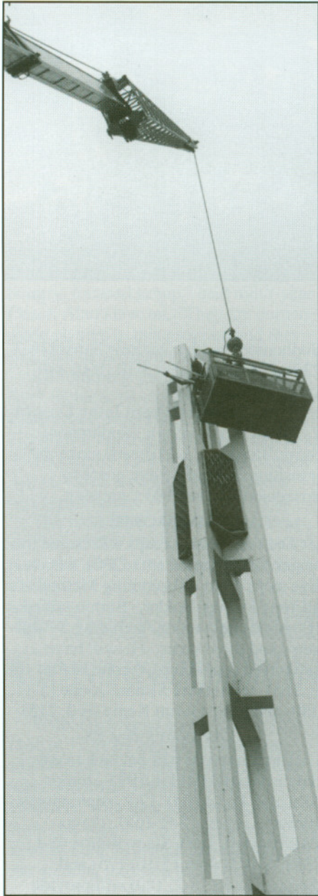
WORKERS FROM DAUGHTRY ELECTRIC REPLACE FLUORESCENT TUBES IN THE CROSS.
