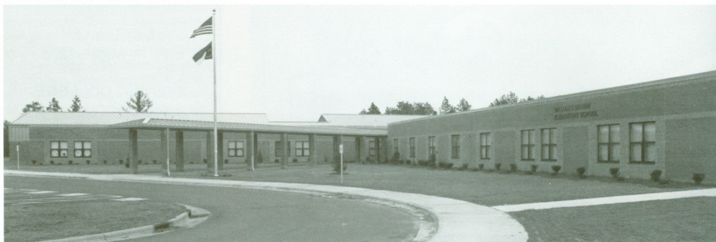
WILLIAM T. BROWN ELEMENTARY SCHOOL IS LOCATED ON A 25-ACRE SITE.
