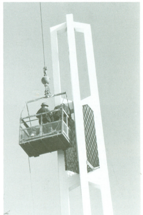
AN ELECTRICIAN INSTALLS NEW SPEAKERS FOR THE CARILLON.
