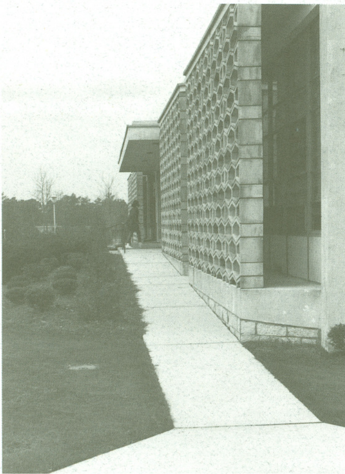
Additions to the College include ramps for the physically challenged so our campus will be accessible to all.
