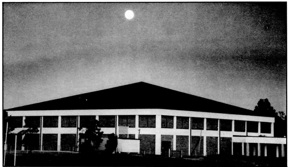
The nearly completed Physical Activities Center (also known affectionately as "The Pyramid") shown at twilight under a rising moon. Photo by Sherry Overton.
