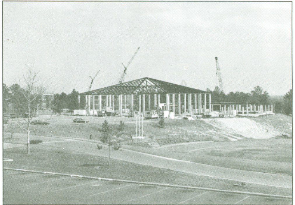
The Physical Activities Center takes shape.
