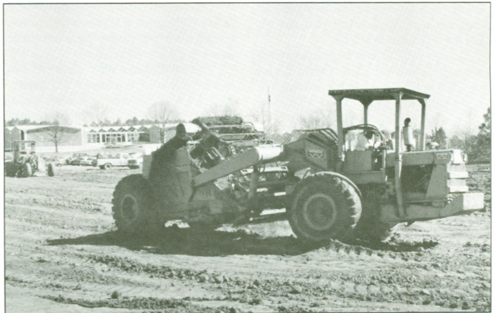
New soccer and field hockey playing fields are now under construction.
