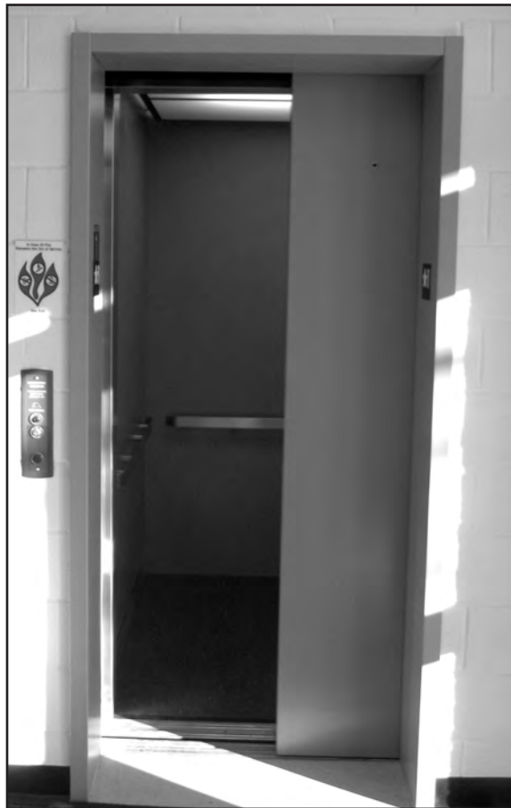
Newly completed elevator in Trustees building. Photo by Jessie Heath.
