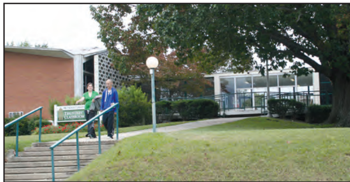
These steps by the parking lot have been a point of contention in recent years. Disabled students must go around the building to the other side to reach sidewalks without steps. Photo by Erik Alegria.
